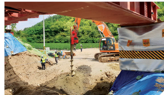
CONFINED SPACE JOB SITE
