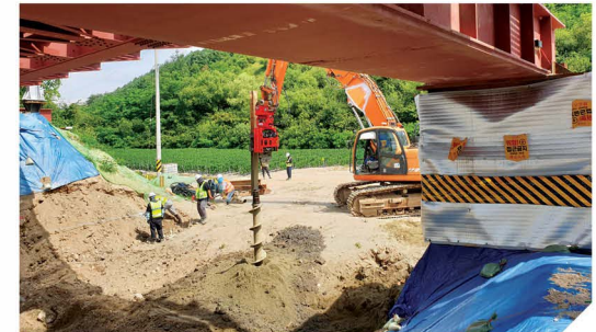
CONFINED SPACE JOB SITE
