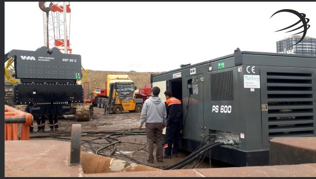
Crane mounted vibratory hammers are operated by seperate hydraulic power packs as there is no hydraulic oil supply in cranes .
